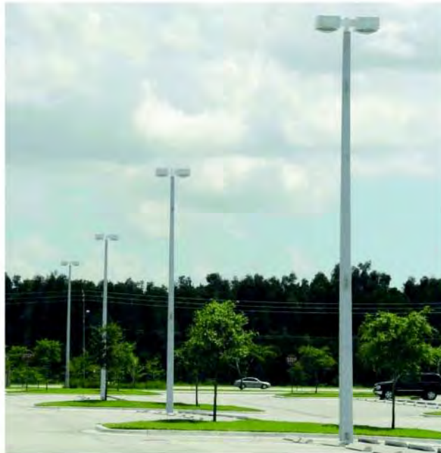
(a) Example Lighting Parking Area
