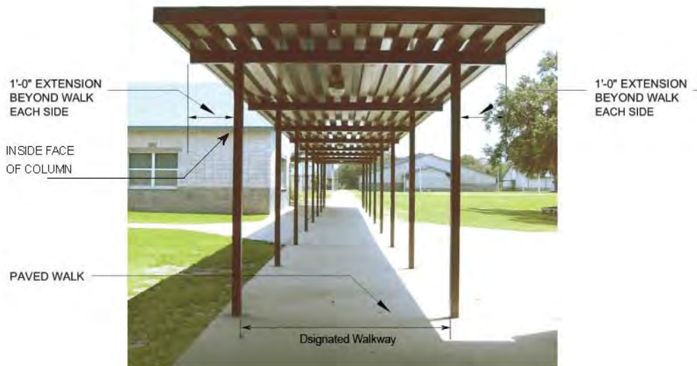
(b) Example covered walkway
